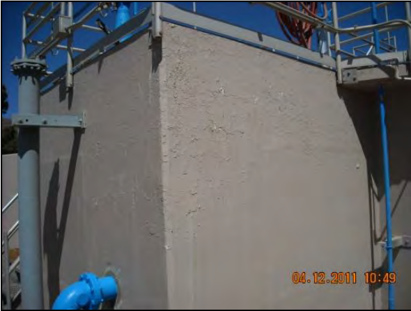
Clarifiers Effluent Box Exterior
