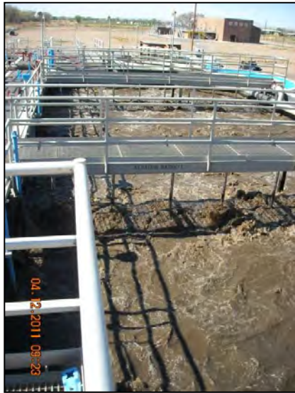
West Aeration Basins
