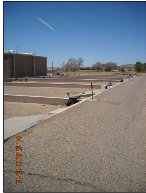
Sand Beds For Sludge Disposal
