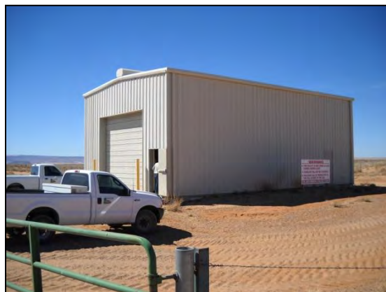
Building Where the Sludge Application Vehicle is Housed
