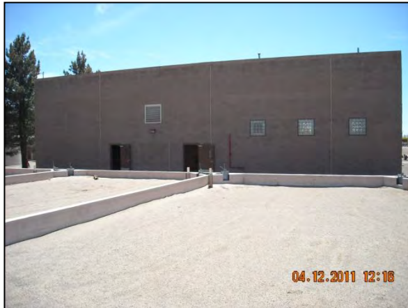
Exterior (North) of the Sludge Handling Bldg.
