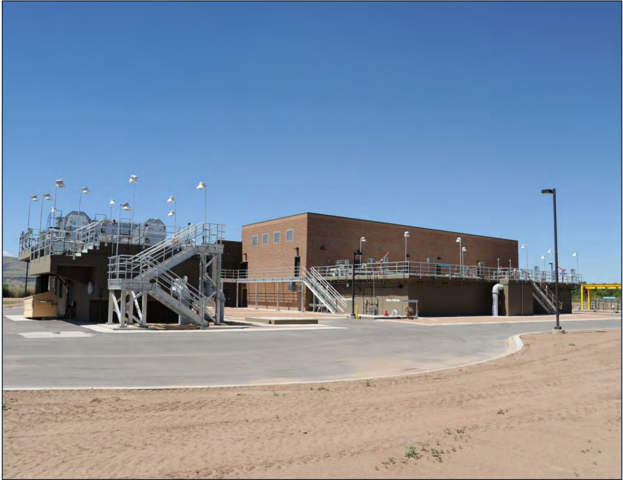
Entrance Works, Pre-Aeration Basins, and MBR Building
