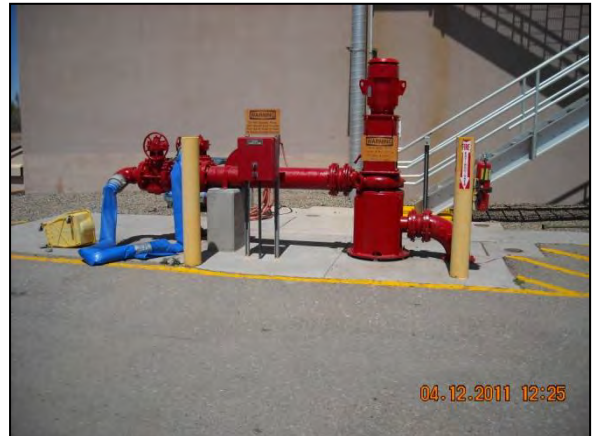
Digested Sludge Pump
