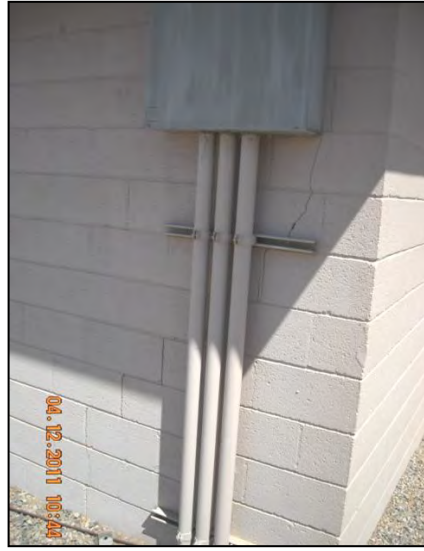
Washwater Room Exterior
