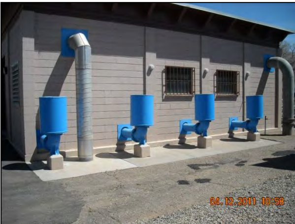
Exterior of the Blowers Room
