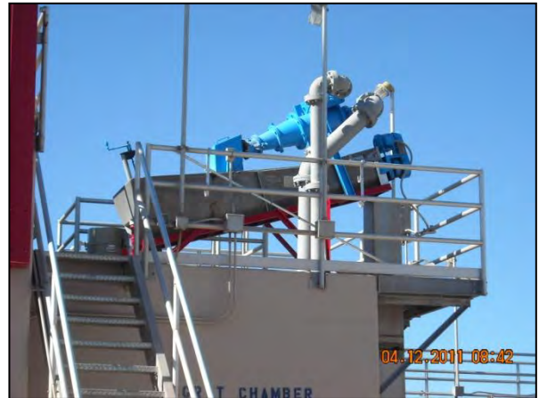
Entrance Works (Hydrogritter on top of the grit chamber)
