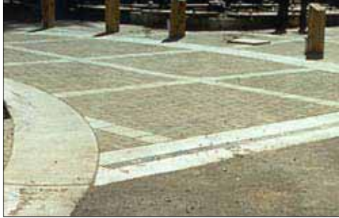
Permeable paving materials reduce surface runoff and treat many pollutants associated with parking lots.
