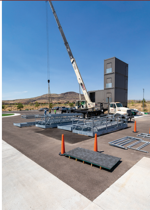
Workers erect new fire department training tower.
